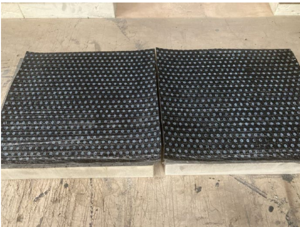
3) Cut the waterproofing base layer using a hook blade
