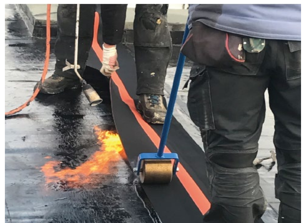
6) Apply pressure using a roller
