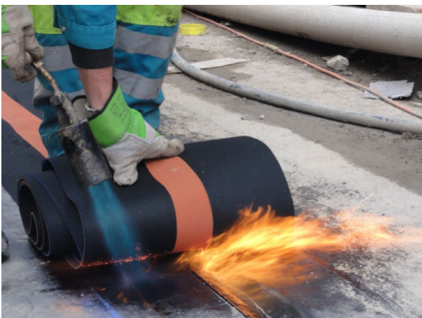
5) Heat the upper face of the waterproofing base layer as the Flexjoint roll is rolled onto the heated bitumen
