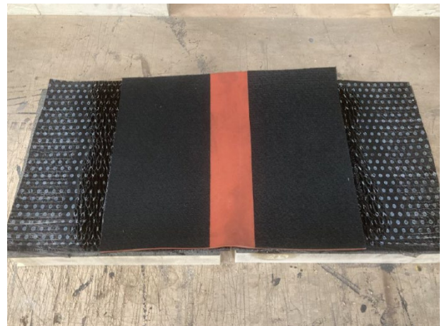
4) Install the Flexjoint over the joint
