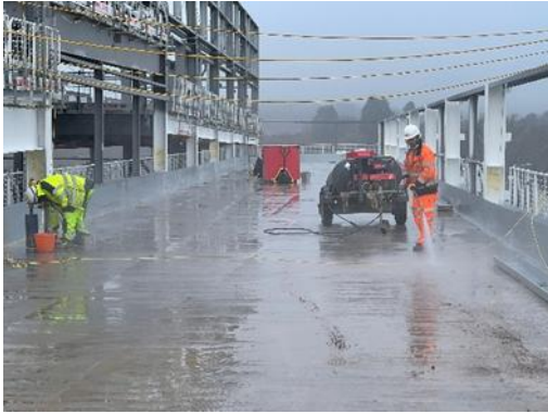
Fig. 6 - Jet Wash Preparation
