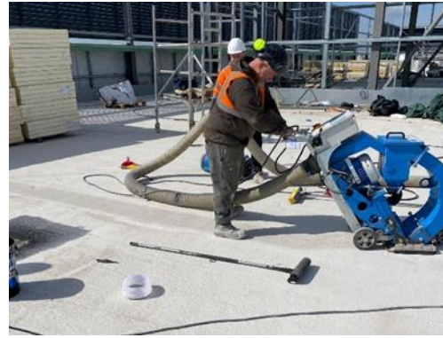
Fig.7 - Mechanical Preparation
